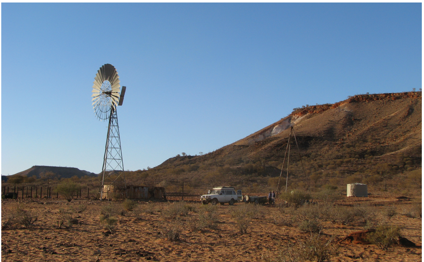
Pumping the water from Cym Bore into the bladder on the trailer. (Libby Sakker)
